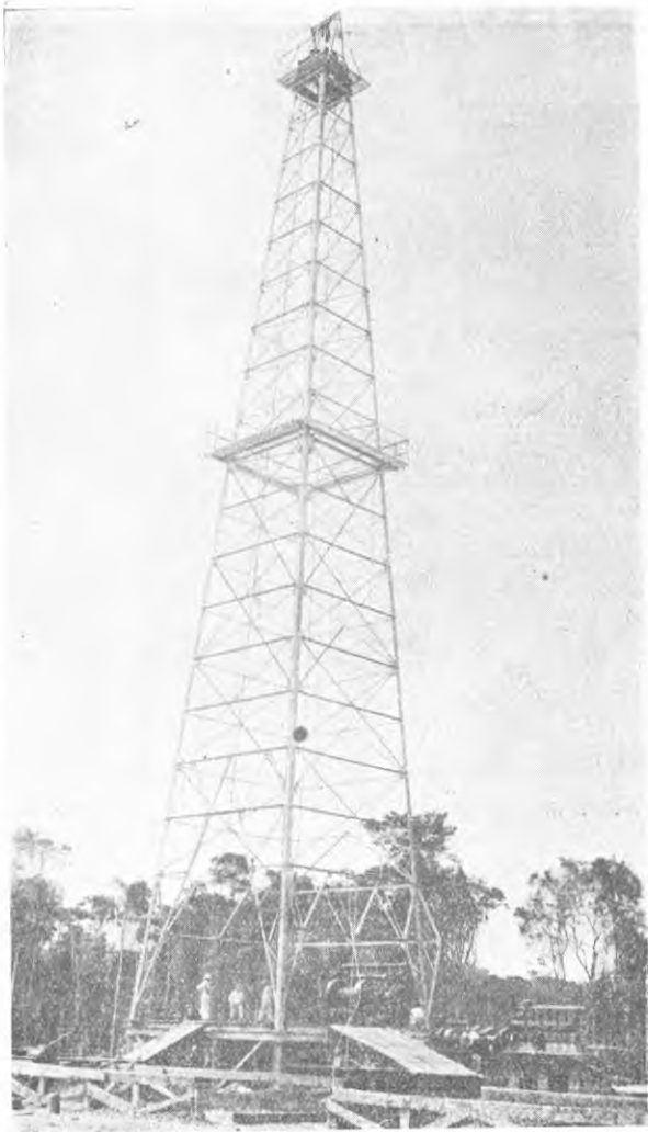
Fig. No. 45.—Socony Narño No. 1 well at the Restrepo Concession, 136-foot tower.
