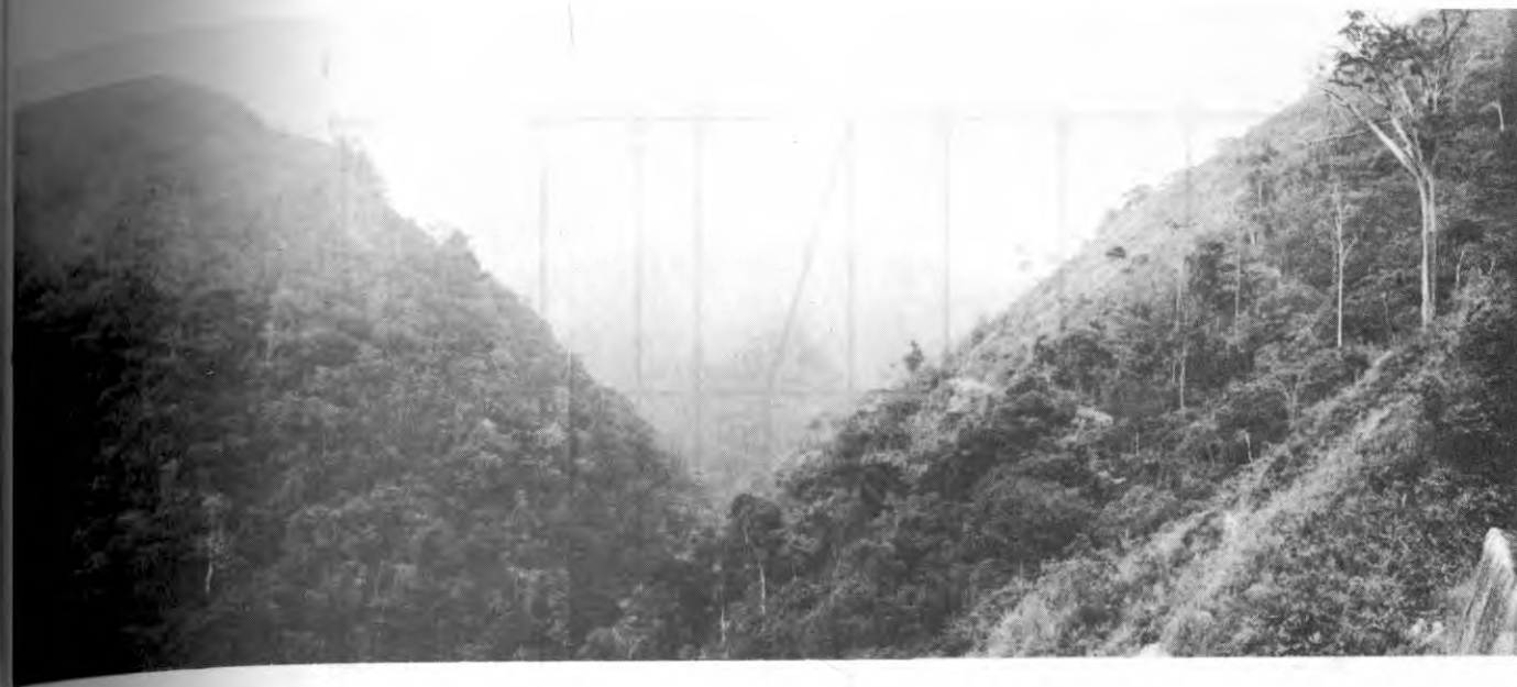
MIEL I DAM SITE, LOOKING UPSTREAM
