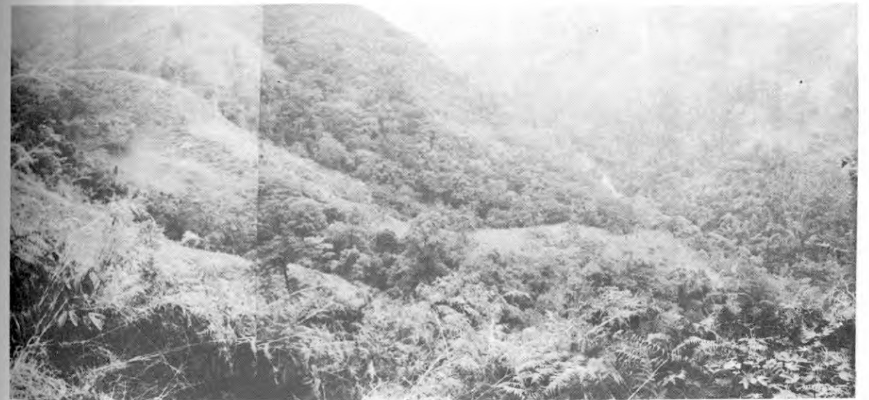
LA FLORIDA SURFACE POWERHOUSE SITE
