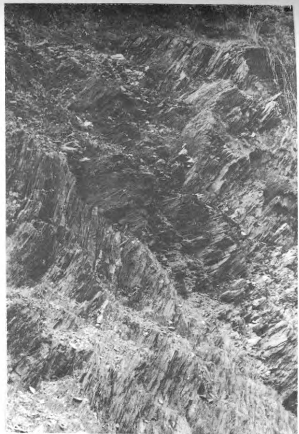
8/9 - Two examples of "toppling failure", overturning of plates of rock accommodated by sliding along the schistosity, in graphitic schist along road cuts near the line of Guarinó tunnel. - Toppling is a characteristic mode of failure in rocks with smooth, regular bedding or schistosity and is facilitated by steep dips and low friction angles.
