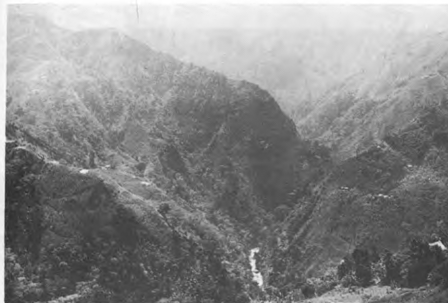
4 - MIEL 2 DAM SITE VIEWED FROM UPSTREAM
