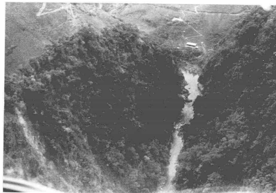
UBALA DAM SITE Downstream end. Temporary field camp is shown
