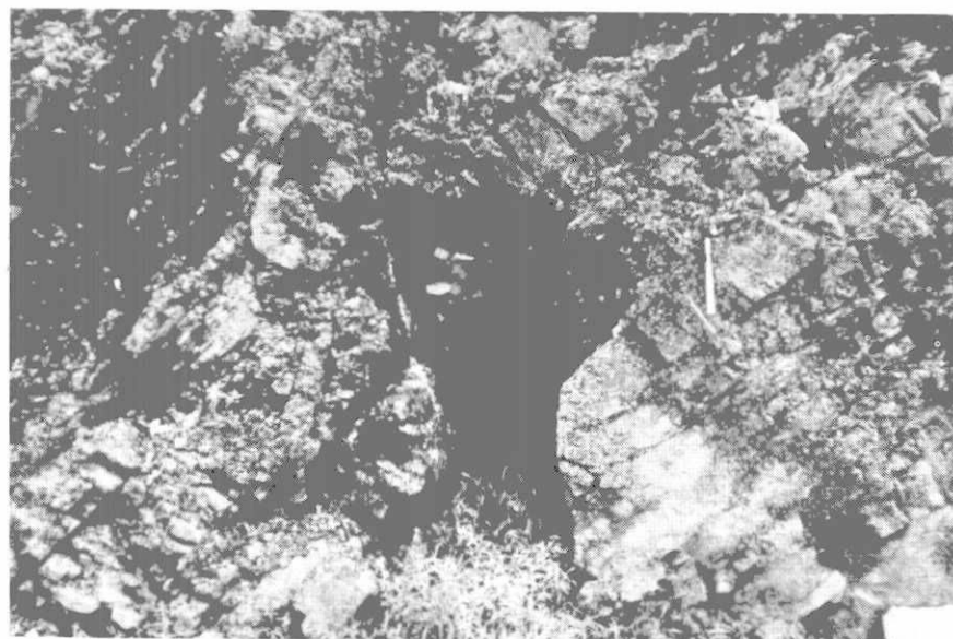
RIGHT, BELOW: CROSS FAULT EXPOSED IN ROAD AT GACHETA DAM SITE — ONE OF A SYSTEM OF SUBPARALLEL FAULTS: SEEMS TO ACT AS A WATER CONDUIT
