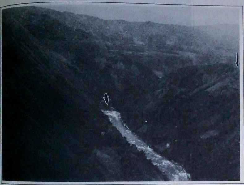
The Guarapas II damsite ( ↓ ) on the Rio Magdalena. A possible branch fault ( ↓ ) of the Magdalena fault passes in the saddle on the left abutment. Note the fill terrace in the background. View is looking south.
